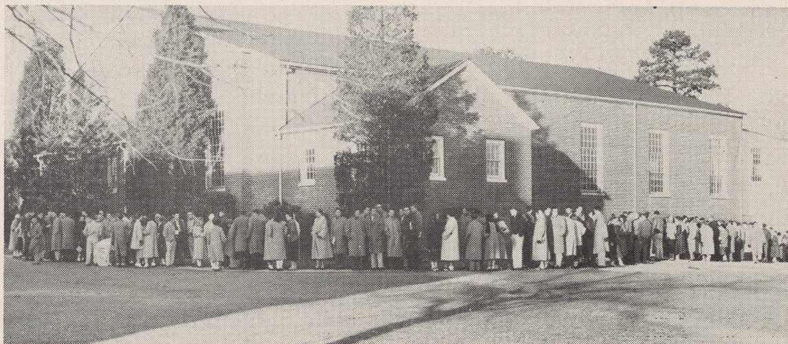
HARRISON GYMNASIUM—COMPLETED IN 1933
