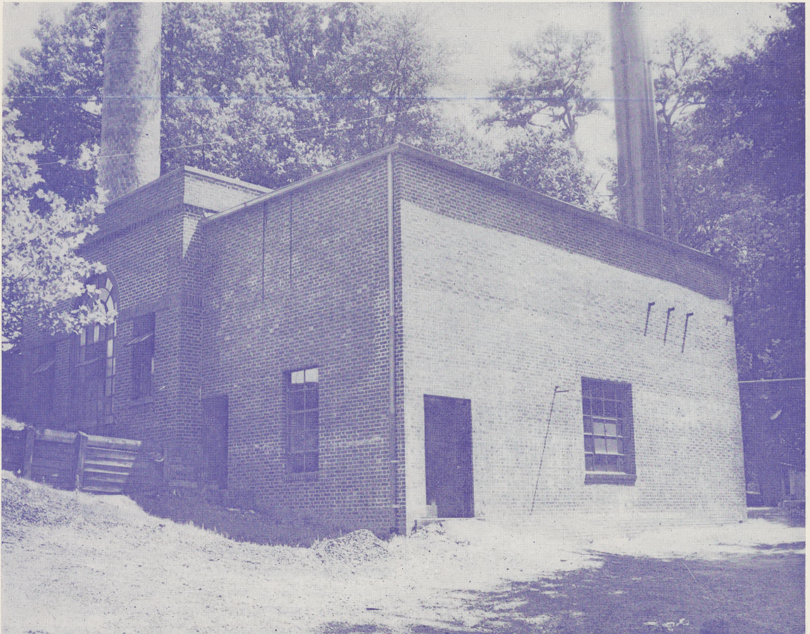
THE NEW ENLARGED HEATING PLANT HOUSING ADDITIONAL AND LARGER BOILERS
