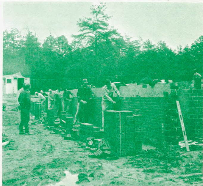
Workmen busy constructing Dormitory
