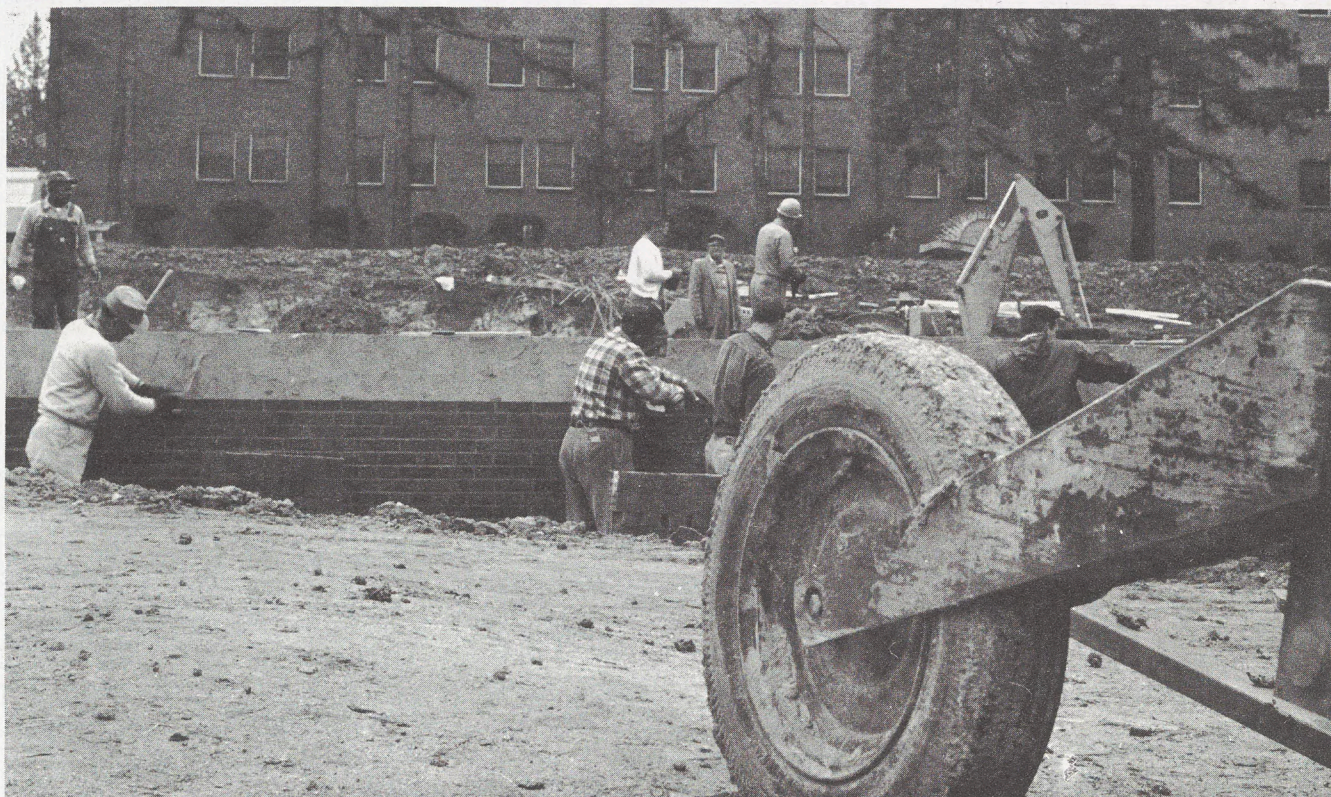
New Dormitory under Construction
