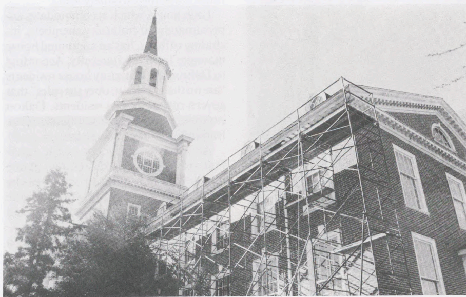
Outside renovation of Roberts Hall has begun.
