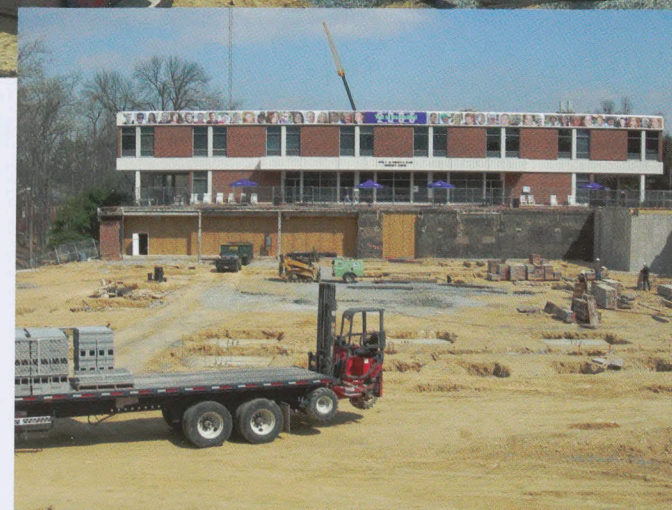
Two opposing views of the Slane Student Wellness Center: above, the massive hole where Memorial Auditorium and Harrison Hall once stood sees a constant parade of construction traffic as the foundation for the new 45,000 square foot building takes shape. Located right in the heart of campus, the building will connect to the current Slane Student Center via a two-story atrium, bringing total square footage of the combined building to 68,000 square feet.
