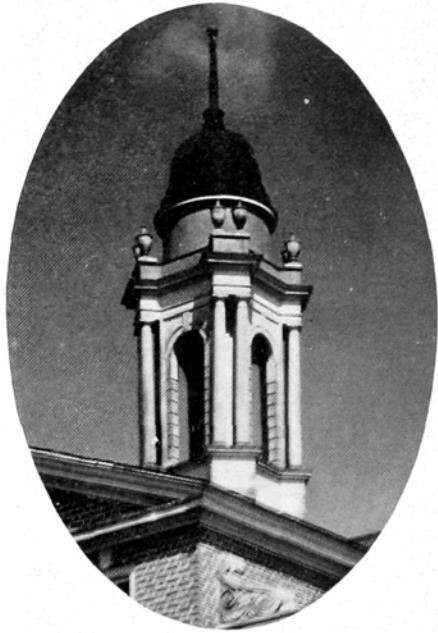
ONE OF THE TOWERS
