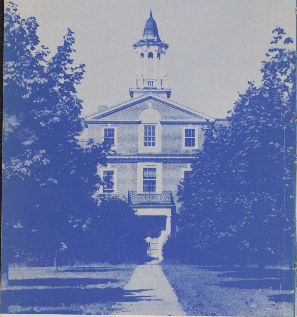
Entrance to one of the Dormitories
