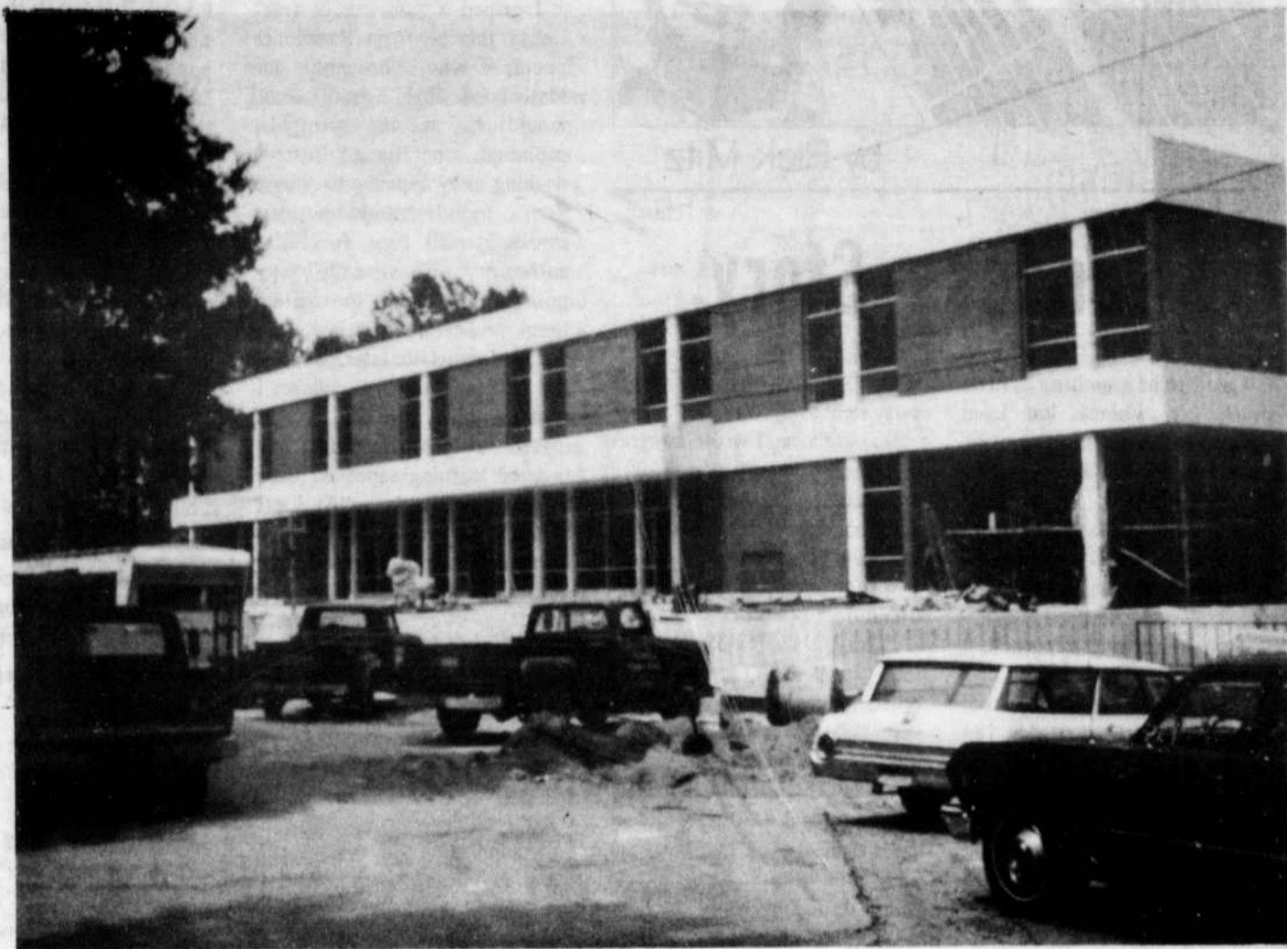
McPherson Student Center under construction
