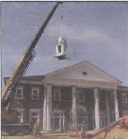
Workers place a steeple on top of the Philips School of Business.
