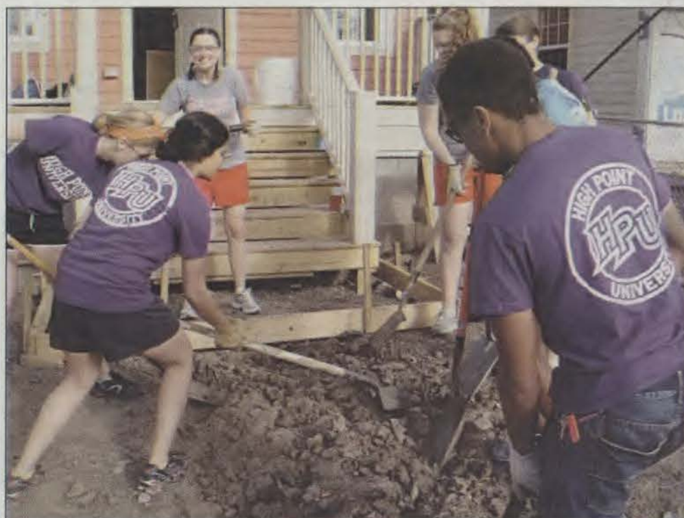
Alpha Phi Omega members break ground to help renovate a home in New Orleans. Photo submitted by Dylan Robinson
